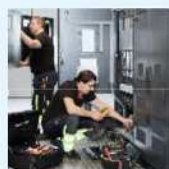
Installation and commissioning
